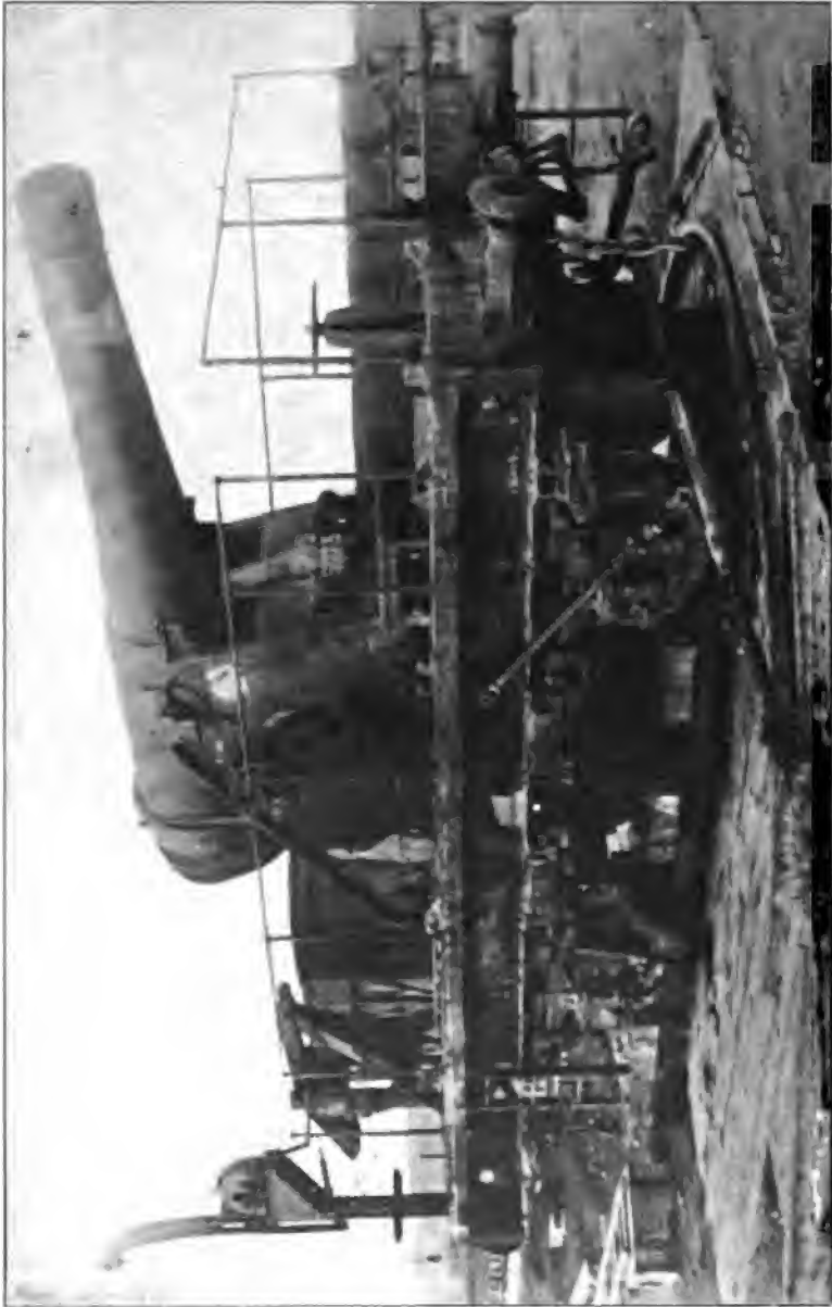
TOP CARRIAGE RECOIL (RUBBER BAND RECUPERATORS) SYSTEM OF THE 190-MM. FRENCH HOWITZER.
